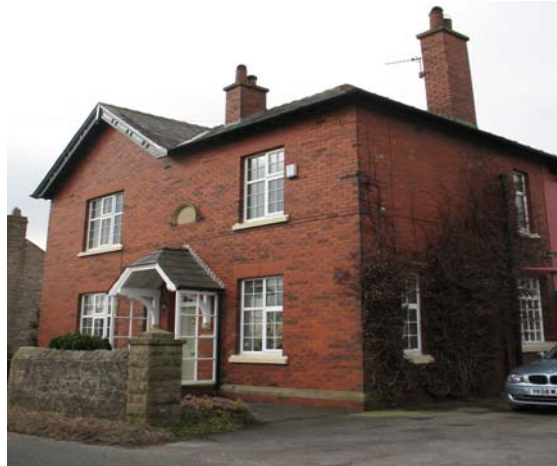
The former Goosnargh Police Station, Button Street
